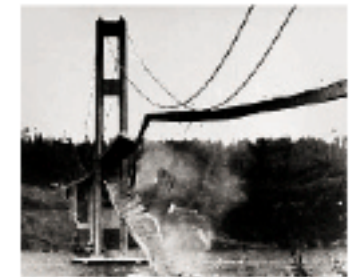
FIGURE 26.12 ▲ In 1940, four months after being completed, the Tacoma Narrows Bridge in the state of Washington was destroyed by a 40-mile-per-hour wind.
